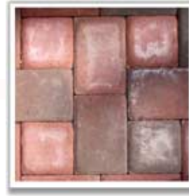
with efflorescence
